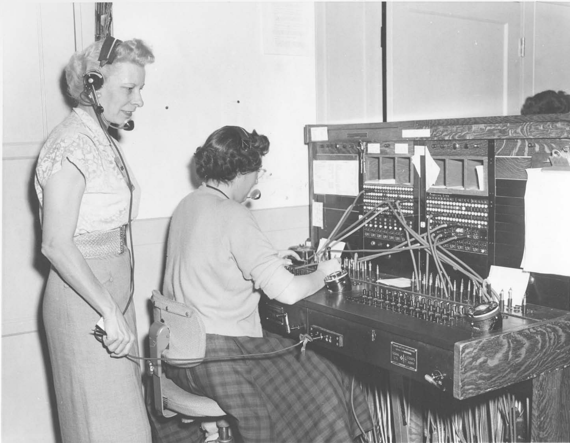
STROMBERG-CARLSON SIGNAL CORPS COMMON BATTERY SWITCHBOARD EDWARDS AIR FORCE BASE, DOUGLAS AIRCRAFT 1955
