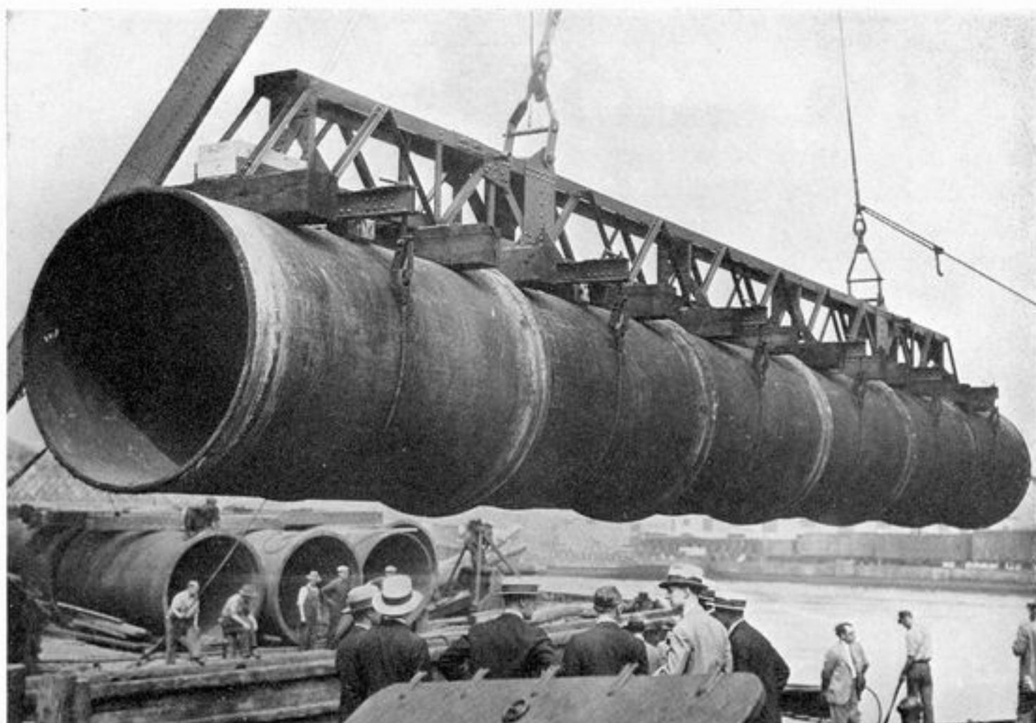
[ Section of giant telephone cable subway being lowered for placement under Harlem River during early 'thirties. ]
