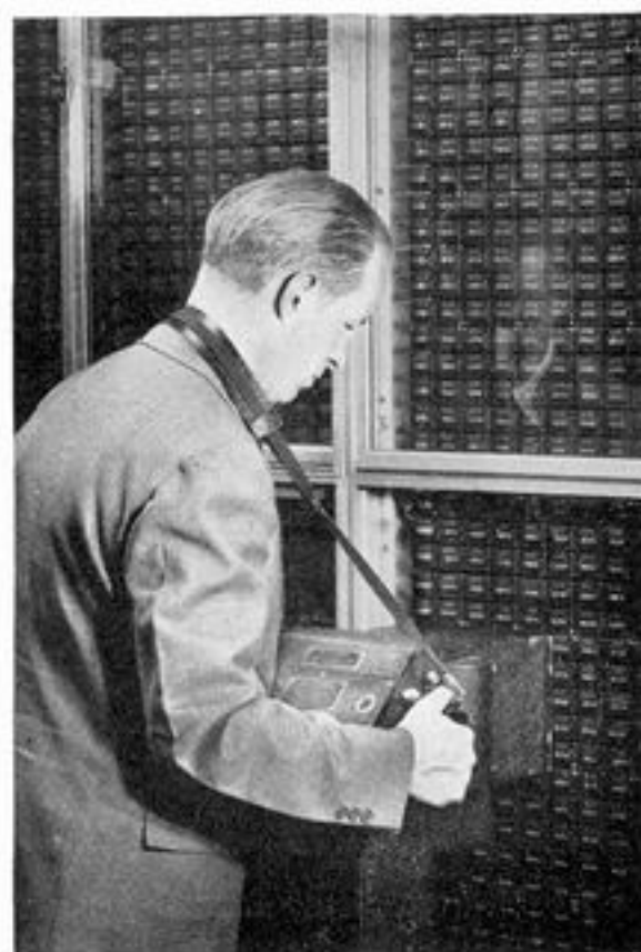
In dial central office, completed local calls are counted automatically by message registers, which are photographed monthly to help clerks in preparing bills.
