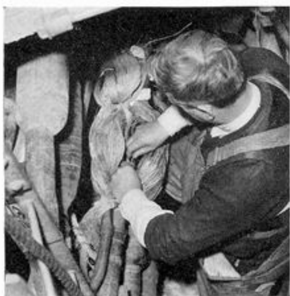
Cable splicer at work in manhole.
