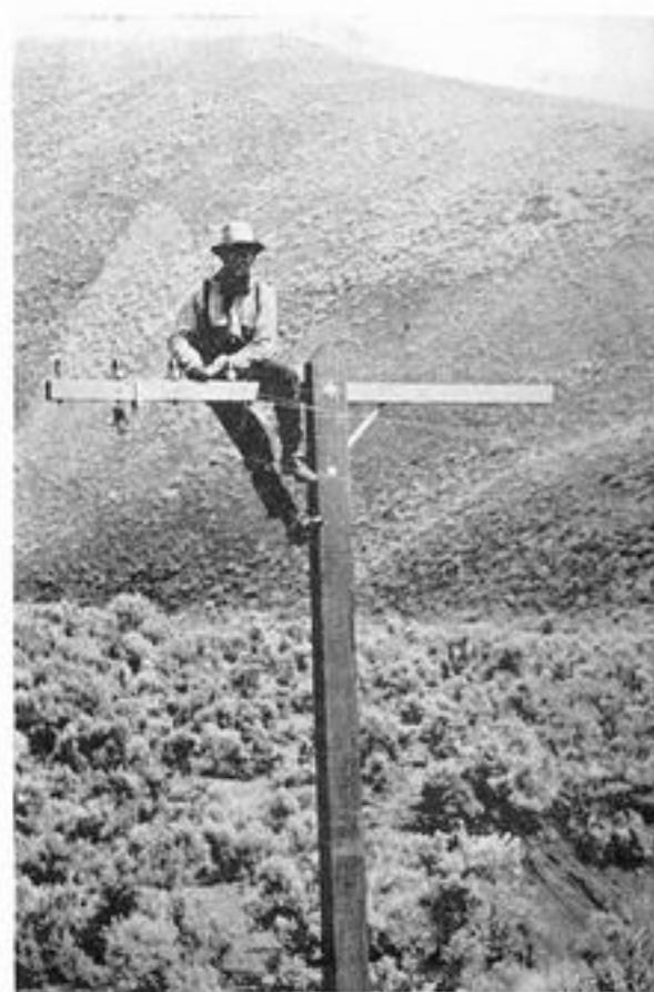
Stringing wires in "bad lands" of the West for the first coast-to-coast telephone line.
