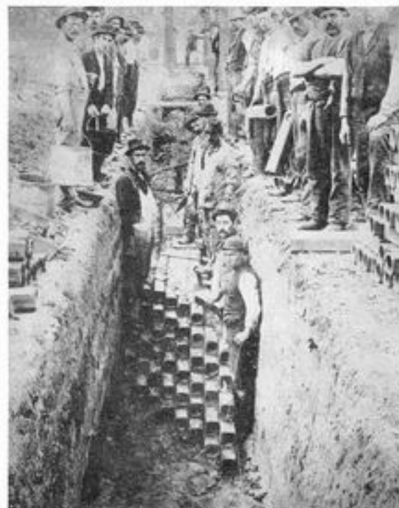
Laying tile conduits for telephone cables in the early nineteen-hundreds.
