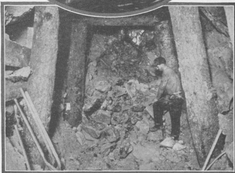
After the blast, the broken rock is taken away, broken into still smaller pieces and processed to obtain the various metals it may contain. The "timbering" is to keep the roof and walls from caving in.
