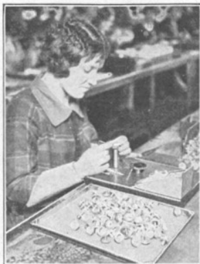
Paper made of linen rags is inserted as an insulator in the transmitter button of the telephone instrument.
