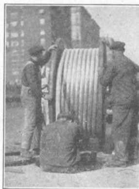
In this familiar scene the telephone wires are being put underground enclosed in their protective sheath of lead and antimony.
