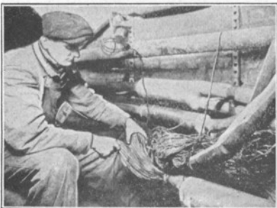
Solder joins the wires in lead covered cables and also joins the lead sheaths where two cables come together, thus preventing moisture from creeping in to injure the insulation.
