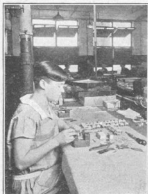
Thin sheets of mica are assembled for the condenser which controls the flow of current and gives the greatest possible clearness to words.
