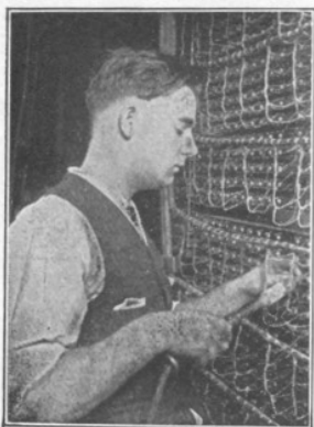
On telephone switchboards in the large central offices (exchanges) there are nearly 4,000,000 soldered joints containing lead.
