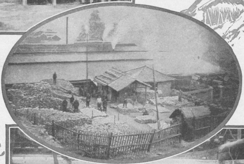
Right—Chinese antimony smelter where the first processes of separating antimony from the ore take place.
