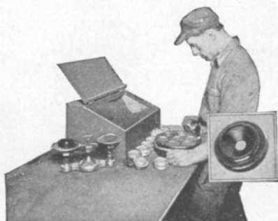
Rubber dust is poured into moulds like that the operator has before him and dies are inserted. When heat and pressure have vulcanized the rubber contents of the mould, receiver caps result, ready to be smoothed to the glass-like surface you have so often felt against your ear.
