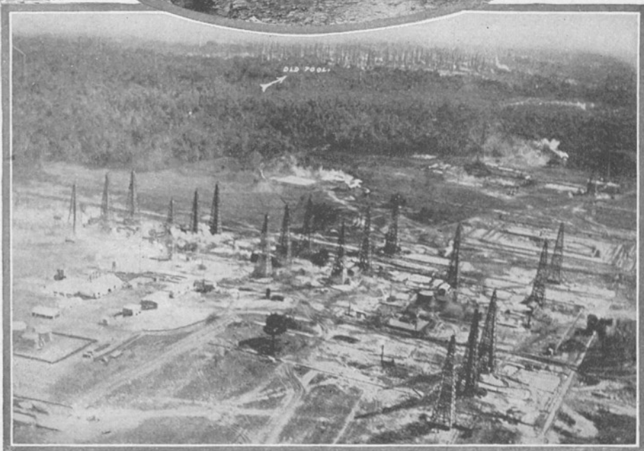
In the United States most asphalt is distilled from petroleum and here is a section of an oil field showing the derricks used to drill for oil.
