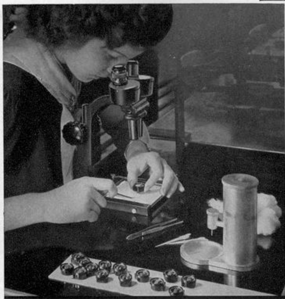
Cleaning magnets of hearing aid receivers.
