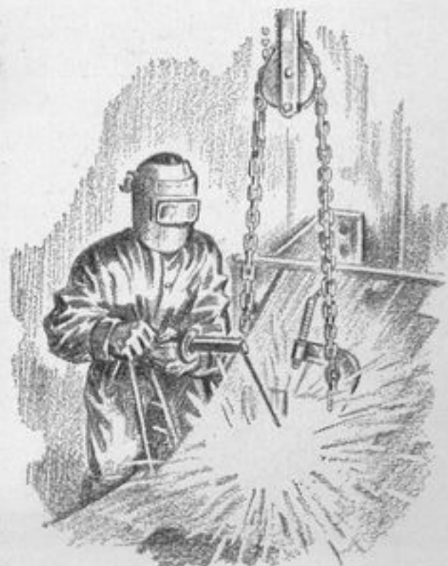
Welding electrically for permanency.
