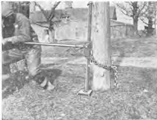
Pulling poles with No. 325—a one-man job
