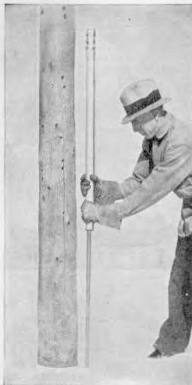
Showing the installation of a 3/4" Ground Rod
