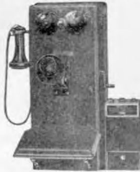
No. 11 Pay Station Attached to N1317 Telephone Set
