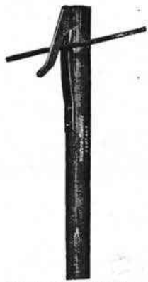
Part of End Section Showing Method of Clamping to Wire No. 4 Line Pole
