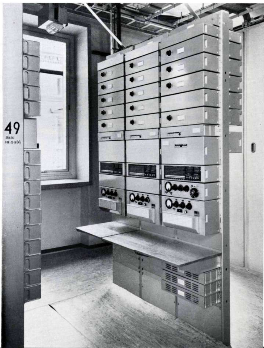
Voice frequency receiver in the trunk exchange
