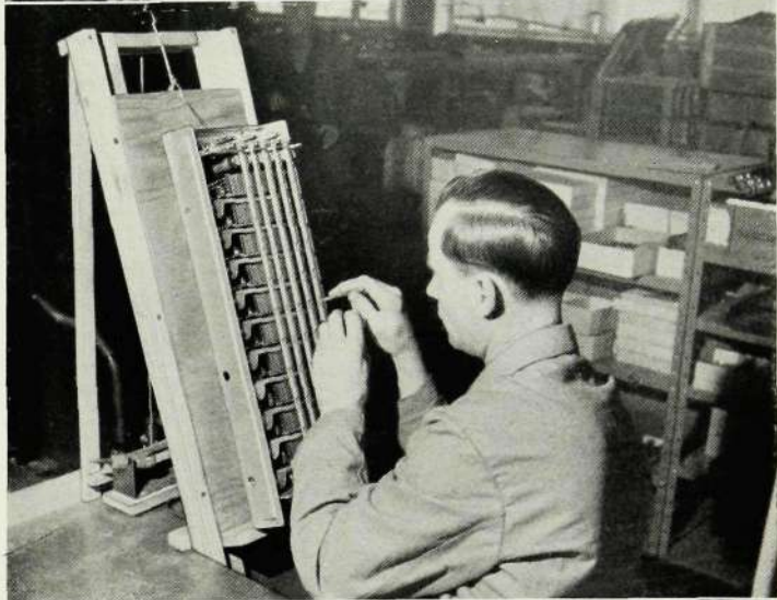
Final adjustment of crossbar switch
